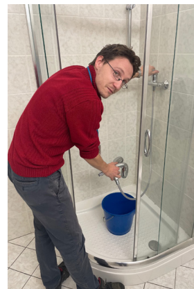
The Energy Scouts tested various watersaving shower heads in the hospital's showers.
