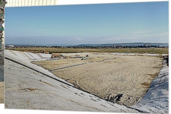
Landfill design, supervision and closure
